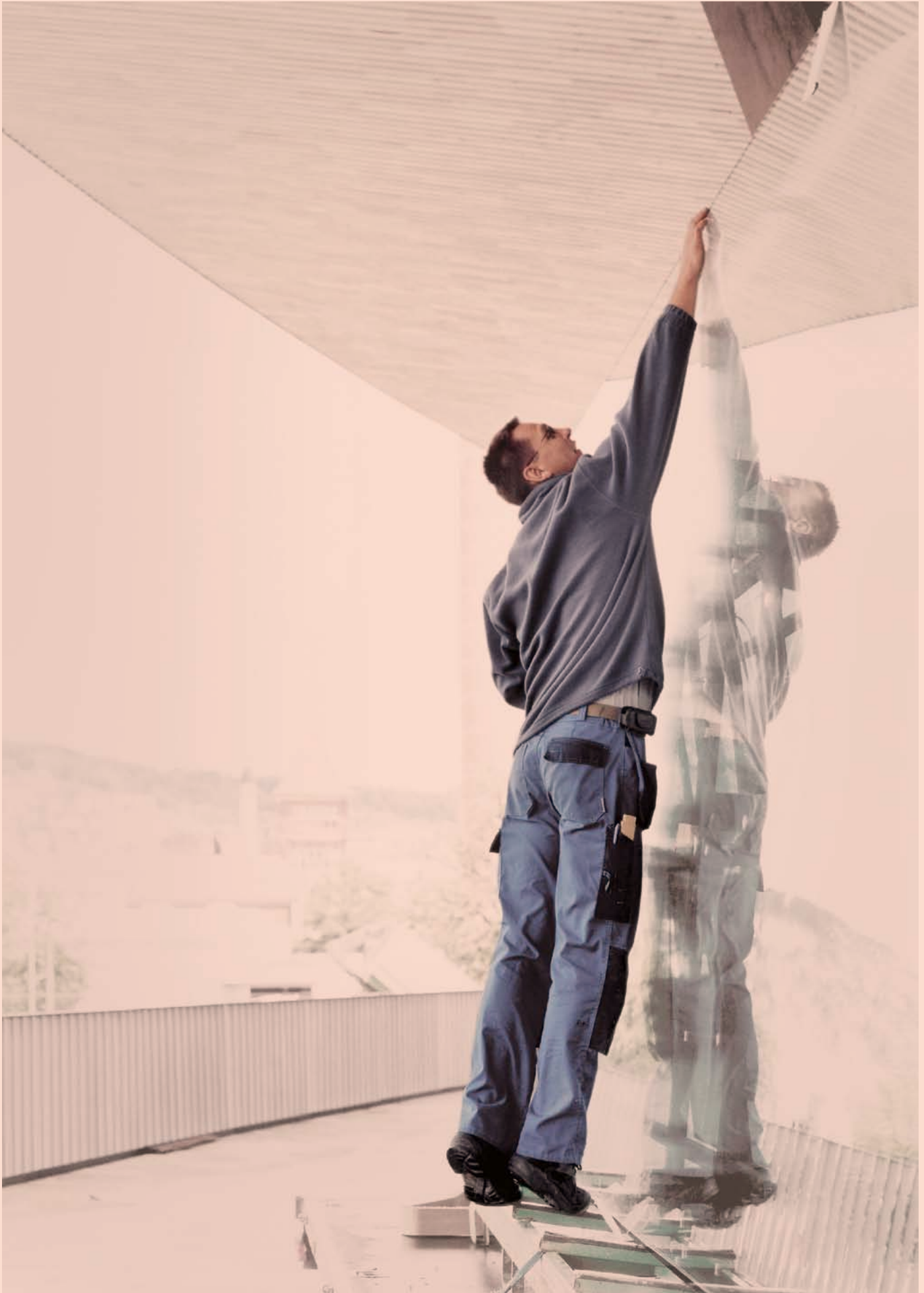
Installation by local partners.
